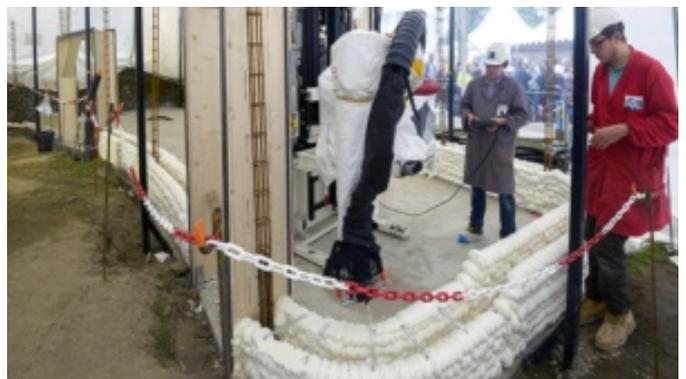
construction, and with its zero waste, raw materials, and decreased transport, the project's ecological footprint was lowered. The project also highlighted how robotic 3D printing technology can lower the risk of musculoskeletal disorders, as construction workers don't have to go up and down scaffolding, and showcased a much lower dependence on good weather conditions for a solid day of construction work.
